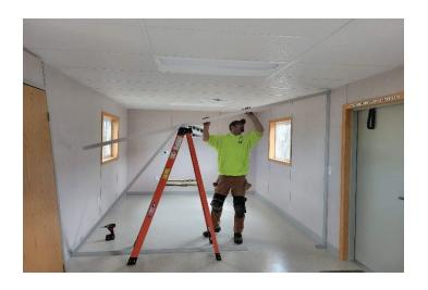
Measure the ceiling wall width and cut the top-track 1/16" short. Place the end of the top-track over the strater track and raise up the other end to the mark on the wall you just made. Secure the top-track to the ceiling every 24".
