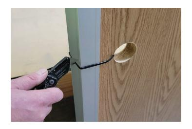
Cut the zip-tie and remove the pastic pipe at the door latch.
