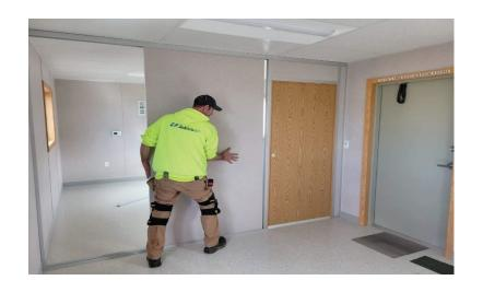
Slide the wall panel into the door panel H-post. Make sure the wall panel is fully within the H-post top and bottom. No screws are needed yet.
