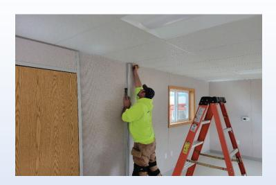
Cut the H-post and the ender-pairs the same as the starter-post, 1/2" shorter than the overall floor to ceiling height. Use the H-post and a level to mark where the top-track will be placed then set aside.
