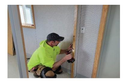
Remove the four jamb screws on the latch side and the four screws on the hinge side.
