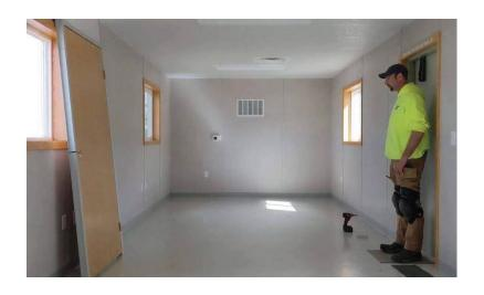
When choosing a location to install the Mod Wall, it is preferable to do so where the main wall stud layout is. Make sure there is no obstruction on the floor or ceiling.
