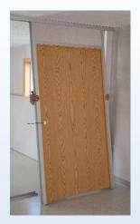
Insert the top of the door panel up into the top-track far enough to get over and into the bottom-track.
