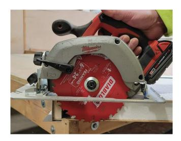
Cut the top of the door panel assembly 1 1/2" shorter than the floor to ceiling height. Us a saw blade with as many teeth as possible to cut through the pre-assembled H-posts and wall panel.
