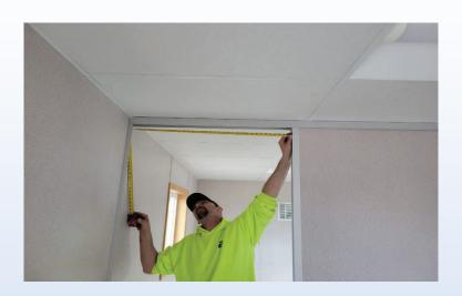
For the last Mod Wall panel, measure over from the outside edge of the H-post to the inside of the ender-pair already installed.
