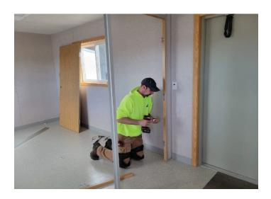
Re-install the four screws on the hinge side jamb. Repeat for the latch side jamb.
