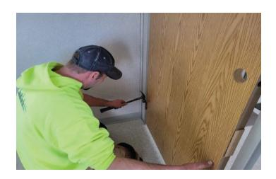
Align the hinges, slip in the hinge-pins and tap down.
