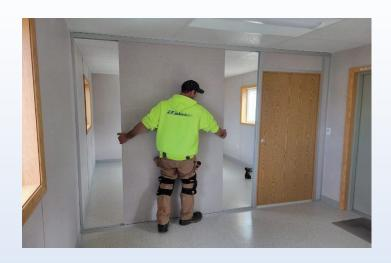
Next is to install a full 48" wide wall panel. Cut the wall panel 1 1/2" shorter than the floor to ceiling height. Insert the top of the wall panel up into the top-track for enough to get over and into the bottom-track.
