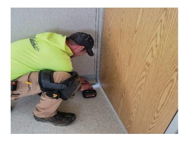
Secure bottom hinge side of door panel H-post to the bottom track.
