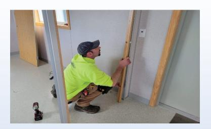
Pull out and down on the bottom of the jamb trim.
