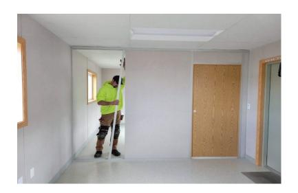
Cut the next H-post from 1/2" shorter than the floor to ceiling height. Insert the H-post into the top-track and over and into bottom-track. Push over and into the wall panel. No screws are needed yet.
