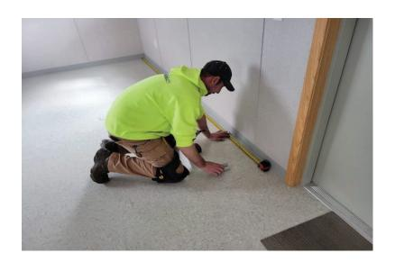
Starting from the door side layout, cut your first piece of bottom track to 5" and secure it to the floor up to the edge of the base. No need to cut the base.
