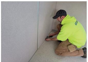
Slide up into the top-track and over and into the bottom-track.
