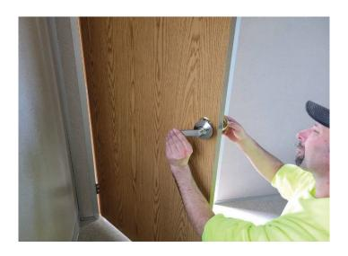
Install lever lockset with screws facing inside the room.
