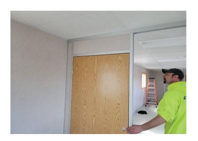
Adjust the door reveal as needed and secure the latch side of the door panel H-post to the bottom-track then the top-track.
