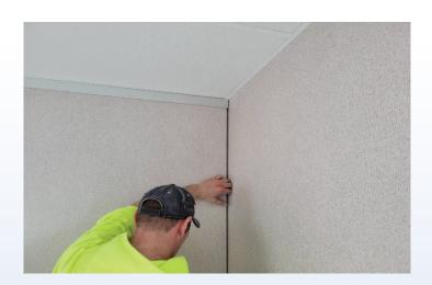
Slide the panel over into the H-post leaving a 3/8" or so gap between the Mod Wall panel and the building wall.
