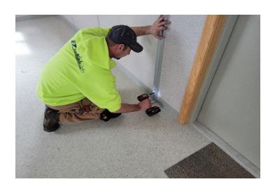
Position the starter post into the bottom track against the wall.
