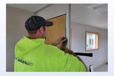
Remove both door hinge pins by tapping them out with a punch and hammer.
