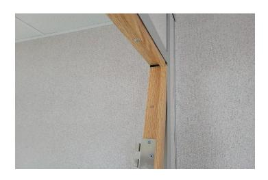
Re-install the jamb trim by sliding the trim up behind the header trim. In this case we want the door to swing in. If we wanted the door to swing out, the door header jamb trim can be removed and turned around.
