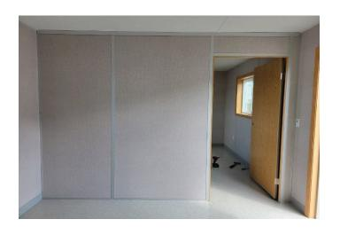
Your wall is just about done! Check and adjust the door if needed and secure the other side now. Open and close the door. If any of the wall panels rattle add additional screws as needed.
