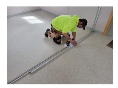
Cut bottom track as measured. Secure by using the H-post to line up the door opening.
