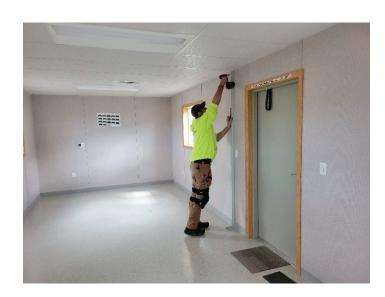
Plumb starter post with a level and secure to the wall with four screws.
